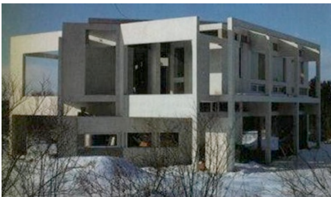
Figura 05 – Casa III (Miller House)
